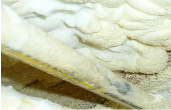
Figure 13. CPVC pipe inside wall covered with PUSF.
